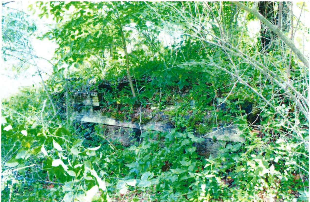
Railroad ties comprising the west edge of Topographic Feature #9, looking northeast
