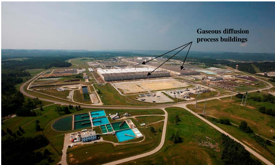
Figure 1.1 The Portsmouth Gaseous Diffusion Plant.
