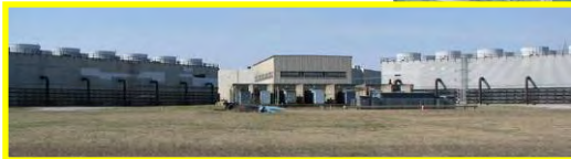
D&D of the X-633 Recirculating Cooling Tower Complex
