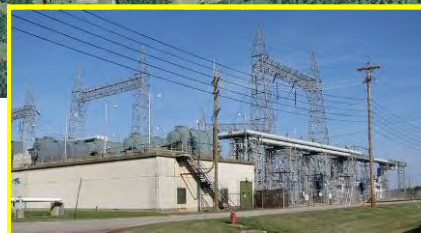
D&D of the X-533 Electrical Switchyard Complex
