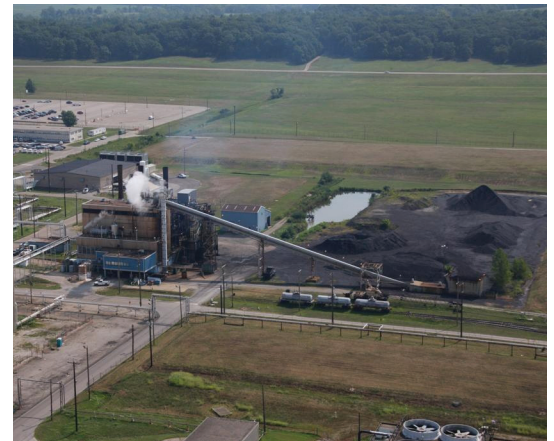
The X-600 Steam Plant is recommended for demolition.
