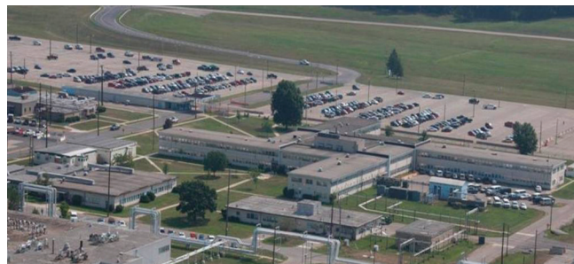
The cafeteria, hospital and administration building are recommended for demolition.
