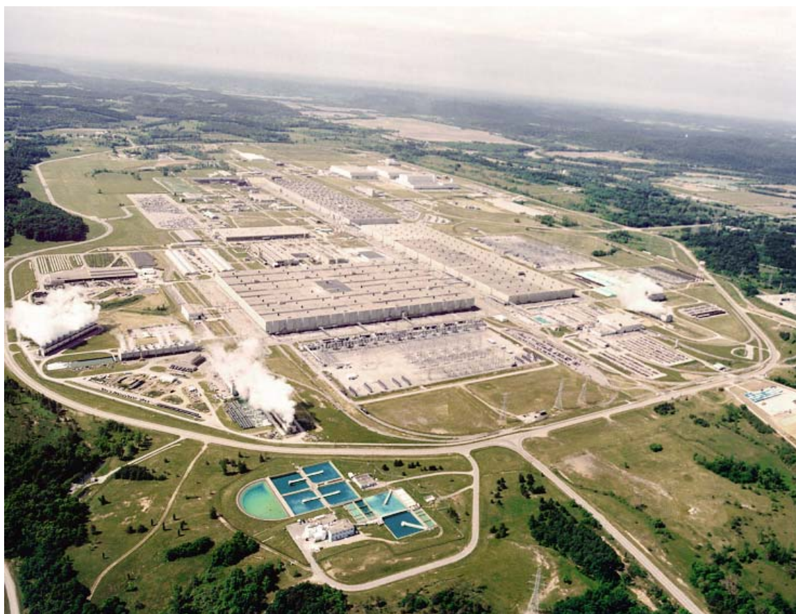
Fig. 1. The Portsmouth Gaseous Diffusion Plant.
