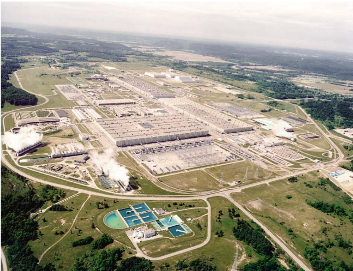
Fig. 1. The Portsmouth Gaseous Diffusion Plant.
