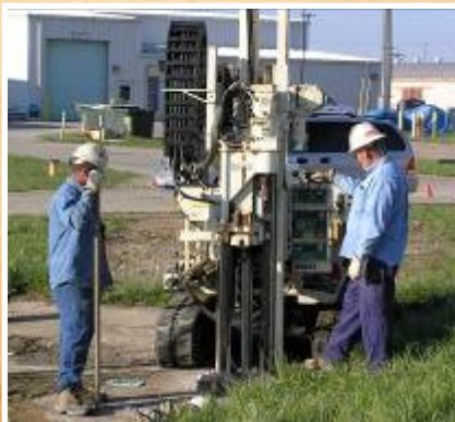
Treatment is injected into the soil at the X-701B plume located on the plant's east side.
