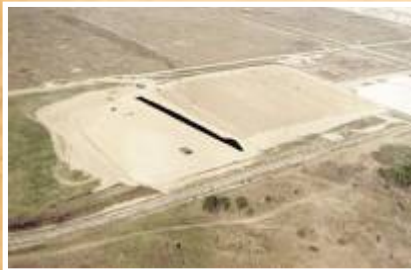
X-749 Low-Level Waste Landfill
