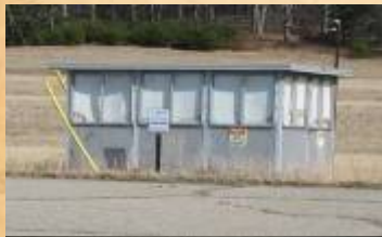
X-230J-8 Environmental Storage Building
