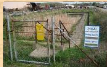
X-342C HF Neutralization Pit
