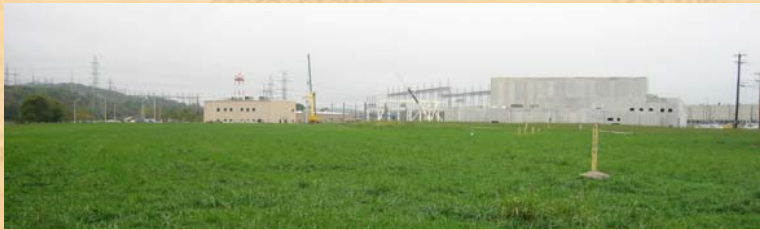
X-616 Liquid Effluent Control Facility
