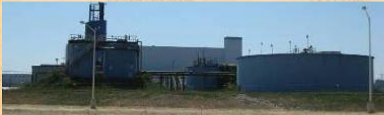
X-616 Liquid Effluent Control Facility
